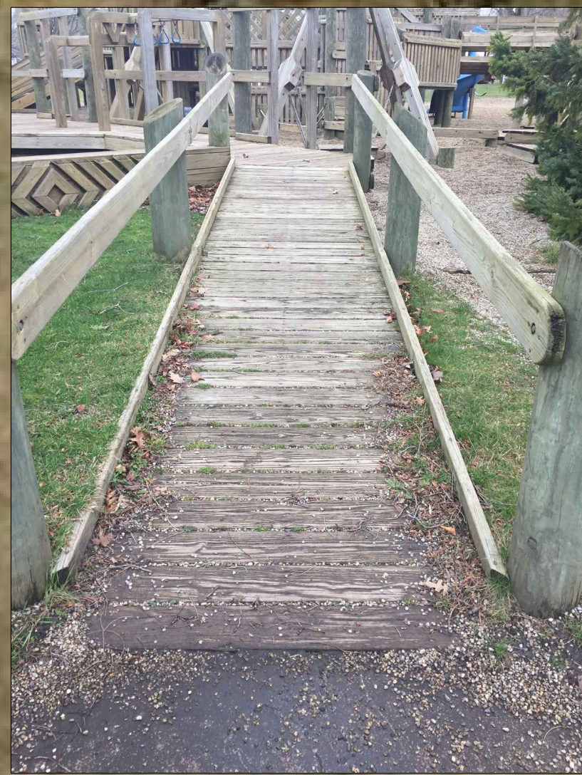
PHOTO OF EXISTING WOOD RAMP
