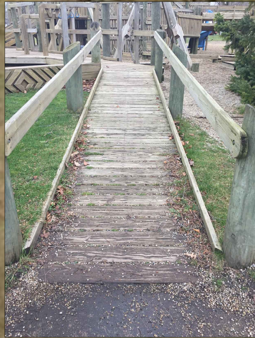
PHOTO OF EXISTING WOOD RAMP
