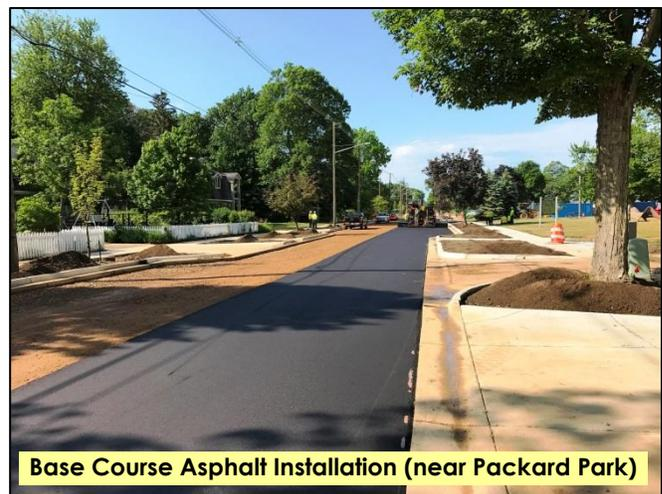
**Tomorrow, June 15<sup>th</sup>**, MPM will be placing the remaining base course asphalt from Webster to Baseline, and the 2<sup>nd</sup> layer of asphalt pavement (leveling course) from Dyckman to Baseline. It should be noted that at the completion of paving operations tomorrow, the asphalt surface will still be approximately 1.5" below the curb level. Residents using their drives should proceed slowly into and out of them until the final asphalt surface is placed.
